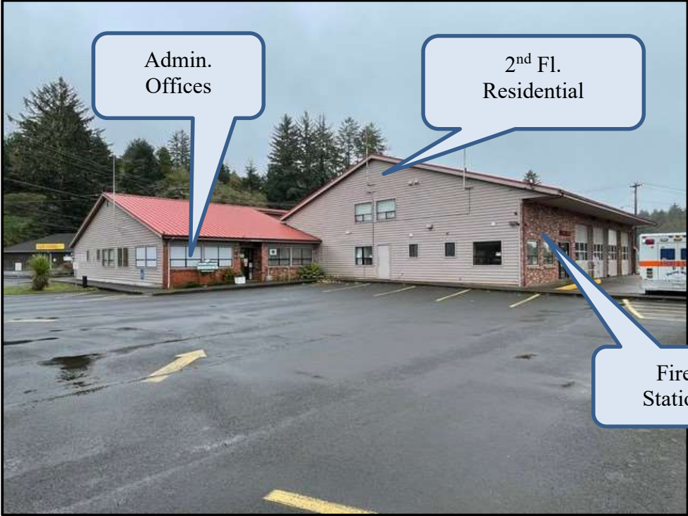
A south-facing overview of the subject site and building.
