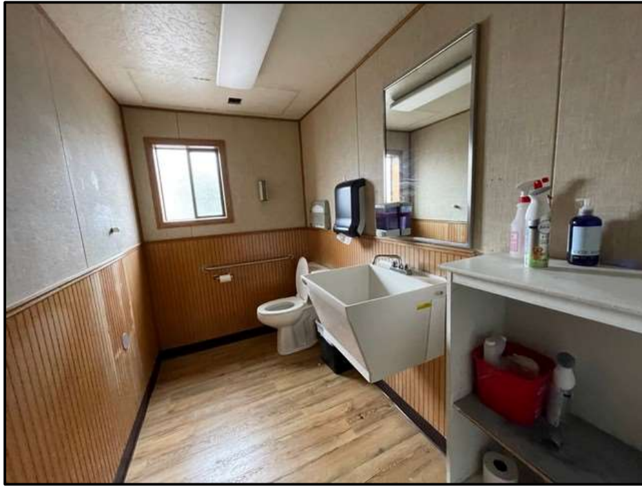
A view of a restroom located on the 2 nd -floor residential space.
