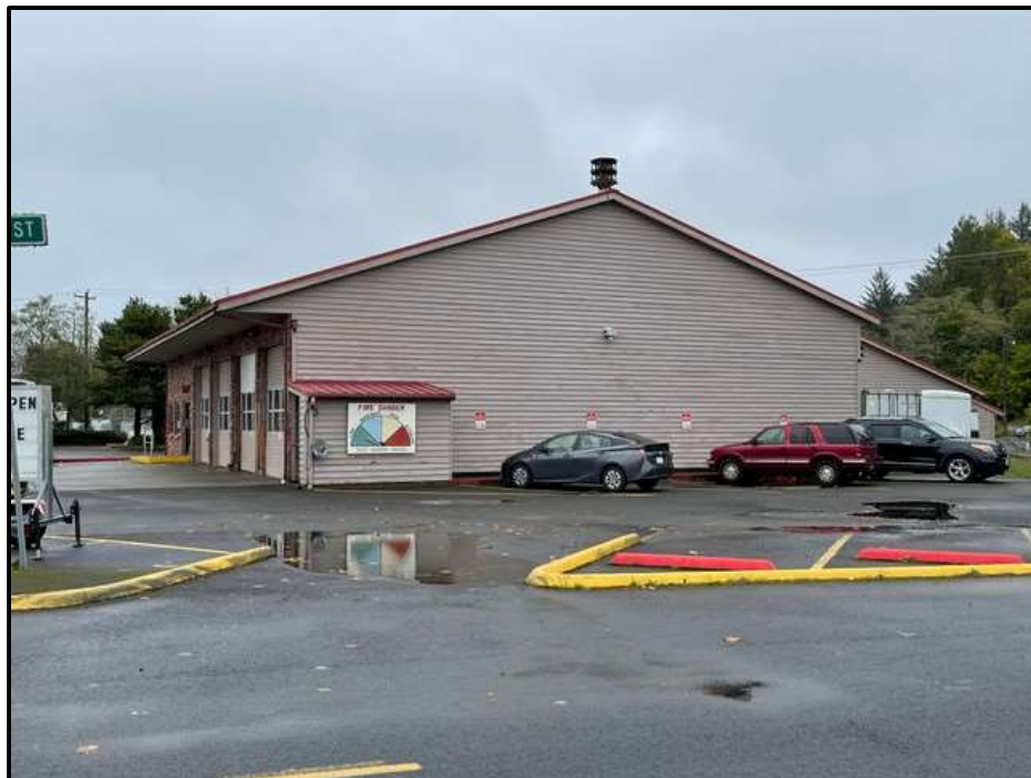
A view of the west and north sides of the fire station.
